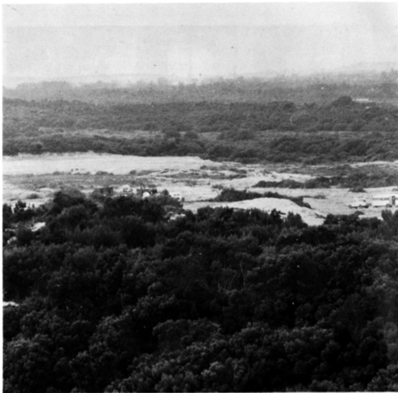
The beginnings of the new Khayalitsha township—dense bush near the Swartklip Road being cleared and levelled for a 1000 site self help scheme. (Cape Times)
